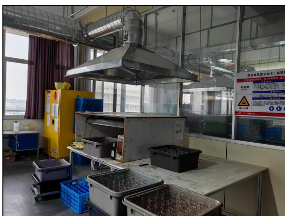
图 4.1-8 粘底、乙醇擦拭工序集气罩
